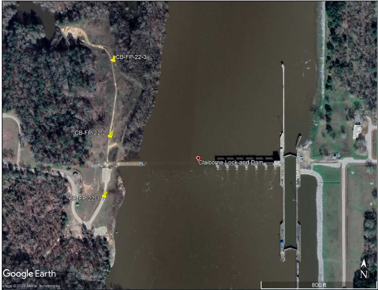
Figure G-10: Proposed geotechnical investigation boring locations requested for Claiborne during this feasibility level study
